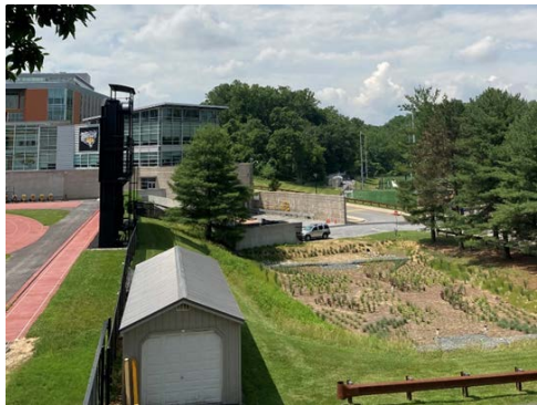
Johnny Unitas Stadium bioretention facility post-construction. Ecotone staff finalized the retrofit with installation of grasses and perennials.
