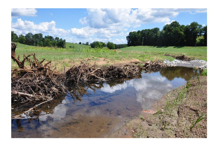
After – As-built toewood structure to reduce shear stress on outer meander banks and provide habitat
