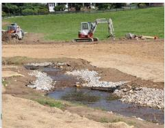
During construction, the invert of the stream was raised and banks graded back to facilitate floodplain reconnection.
