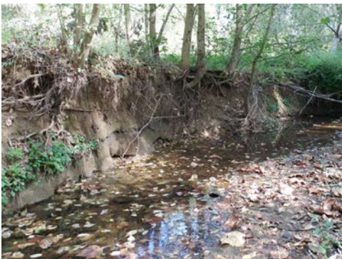
Prior to restoration, North Branch Bennett Creek and its tributaries were disconnected from the floodplain, with vertical banks showing vegetative overhang and exposed roots.
