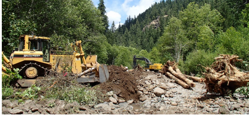
Figure 3: Berm material being pushed into the incised mainstem channel.
