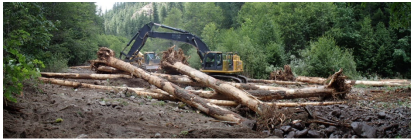
Figure 4: Typical logjam construction.
