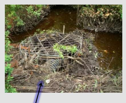
Note the extreme activity at this cage. The cage was only 6' from the culvert (dam site). However, the culvert remained open and functioning. Road flooding has been eliminated.
