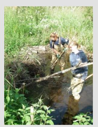
Notch dam slightly below target pond levels, removing wood and debris that would interfere with the pipe installation. Make sure that the pond water is not released too rapidly to prevent downstream
