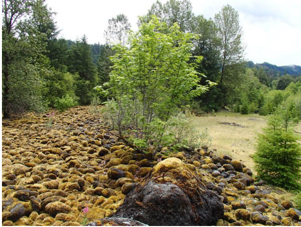
Photos B-1 and B-2. Riprap adjacent to SF McKenzie River inhibiting floodplain interaction.
