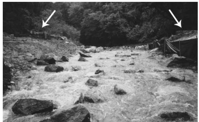
Figure 2. Example of a dam removal approximately one week following removal. View is facing upstream from within the area of the removed dam. White arrows mark the remaining abutments of the original dam face. The channel has been created by removing impounded sediment to match the shape of a downstream reference reach. Cobble substrate placed on the streambed will resist erosion in accordance with sediment transport theory. The banks are cut to a stable slope, stabilized at the base with large cobbles, and seeded with native vegetation. Compare with the channel in figure 1b.
