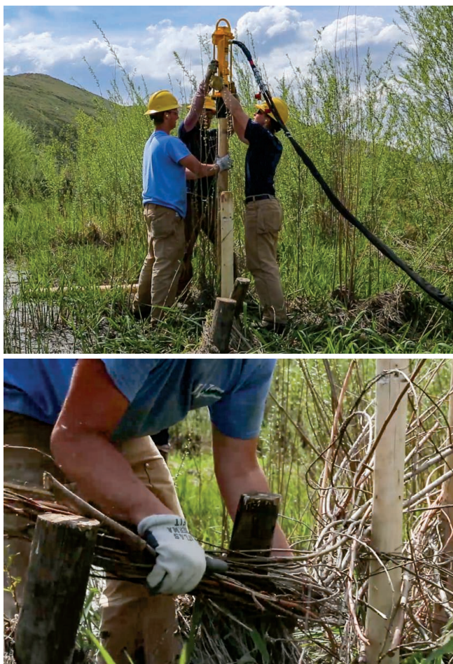
On Oregon's Bridge Creek, researchers create an artificial beaver dam by pounding logs into the stream bed (top), then weaving a lattice of sticks (bottom).
