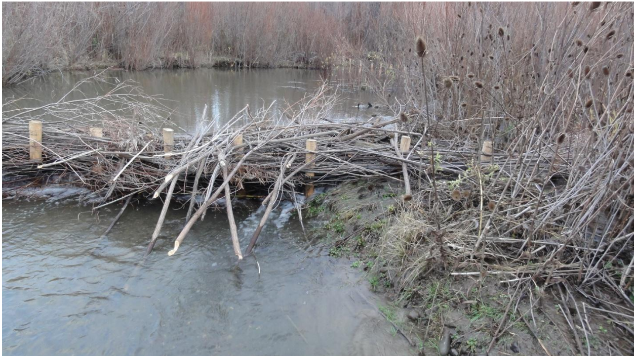
Figure 11. A post line with wicker weave is similar to a starter dam, but acts more like a weir in that water is allowed to flow through the willow branches such that low flows are not over topping the structure and the woven branches may not extend to the top of the posts. These may naturally seal up by trapping sediment and organic material moving downstream or they may be utilized by beaver. Note that beaver have started to colonize this PLWW, as evidenced by the chewed stems on the right of the photograph, aligned parallel to the flow.
