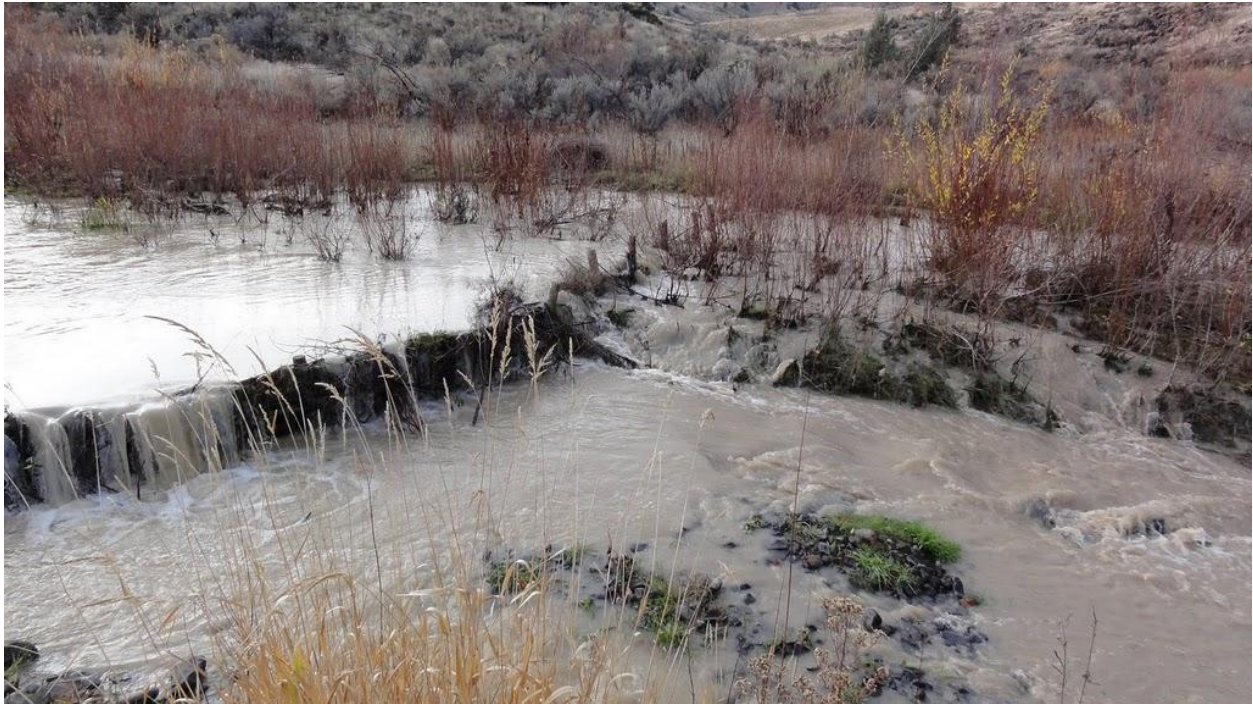
Figure 10. A typical starter dam (SF-17 at Sunflower) with willow branches woven between vertical posts and the back side sealed with rock and clay. Note the dam height is sufficient to divert flow onto the RL terrace, mimicking a stable beaver dam.
