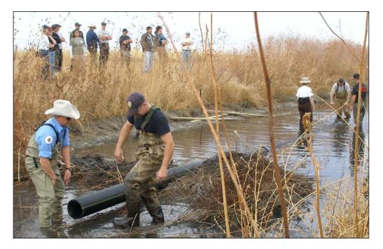
This relatively inexpensive and easily built beaver deceiver immediately lowered the water level and allowed the beavers to stay in the area.
